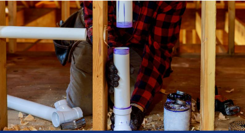
off the riser are rigidly constrained. This induces stress onto the connection and it may eventually fail.
